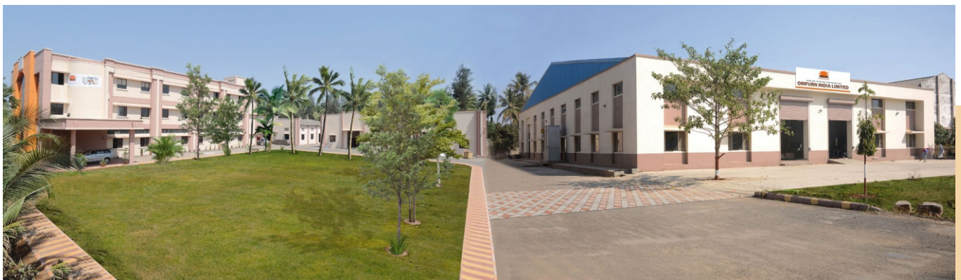
The factory at Umbergaon, spread over 10,220 sq.mtrs. built up area standing on 15,000 sq.mtrs. plot
